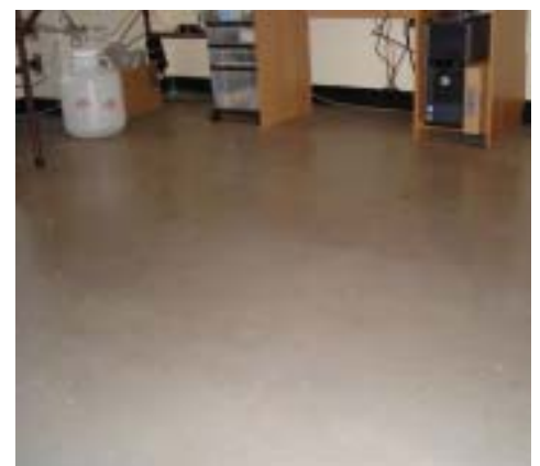
Concrete Floor After
