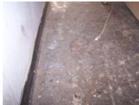
Concrete Floor Before
